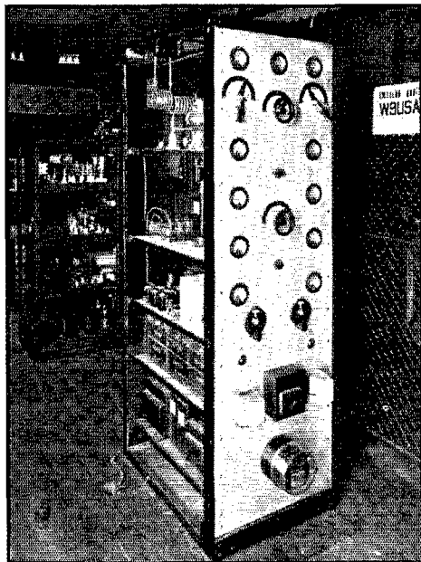
THE MAIN TRANSMITTER—W9USA
